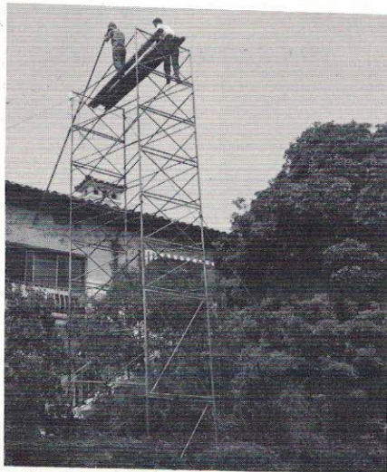
Plumb loco plumbers build tower of Babel!
